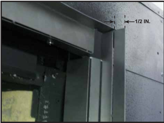
Figure 13.4 Finishing Templates Bends - Inoperable (Fixed) Doors
